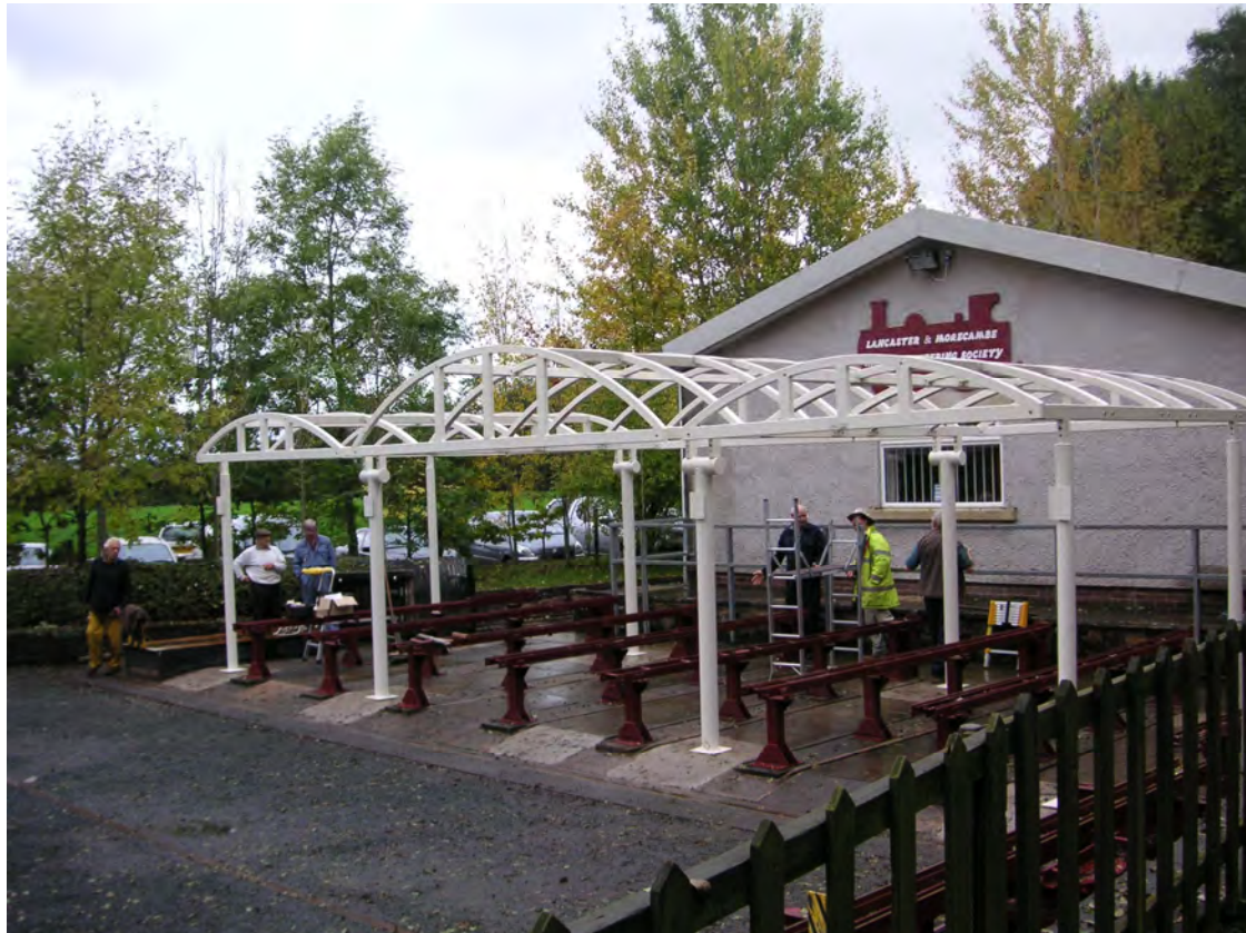
THE NEW STEAMING BAY ROOF TAKING SHAPE
