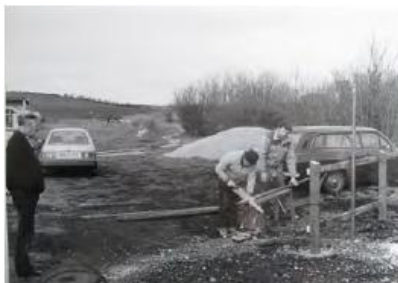
Track laying at Steamtown 1985
