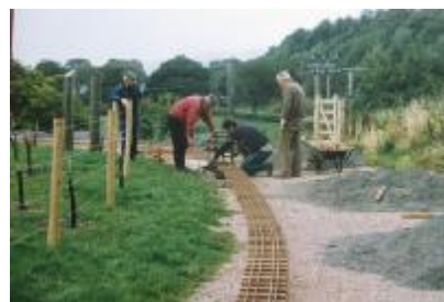
Track Laying at Cinderbarrow
