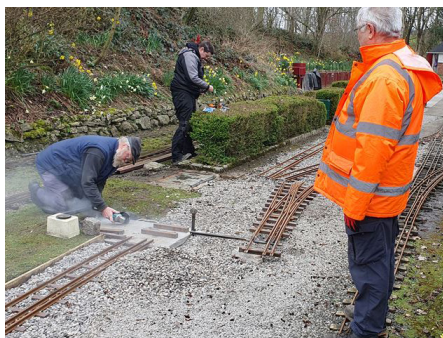
Final adjustments are made to points for the new track
